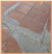
NOTE that Revestech waterproofing system is completely watertight and non-porous. For this reason, it is of utmost importance to follow the recommended steps to lay and install the finished flooring correctly and prevent such phenomenon as efflorescence.
