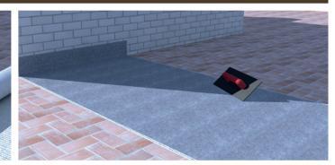
1. Check stability of the substrate and clean surface. Then apply C2 S1/S2 tile 2. Press the membrane firmly onto the substrate with the help of the trowel, making adhesive with 4/6 mm notched trowel. Apply the adhesive in small sections to sure to remove any air that may have been generated. NOTE: once installed, check
