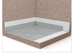
1. Clean well removing all existing residues on the substrate. Apply C2 S1/S2 tile adhesive using a 4/6 mm notched trowel. Spread the ECODRY50 membrane over the adhesive, rising a minimum of 10 cm on the wall. Check that the membrane is well extended, with the help of the trowel, remove any air that may have been generated. Form the corners by folding the membrane. For a perfect finish use the precast items ECODRY50 CORNERIN and ECODRY50 CORNEROUT.
