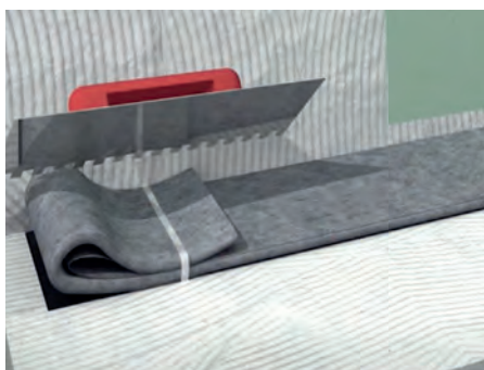
11. Adhere the ECODRY BAND heat-sealed to the LINEAR / SUMI LEVEL with C2 S1/S2 adhesive on meeting points and slopes.
