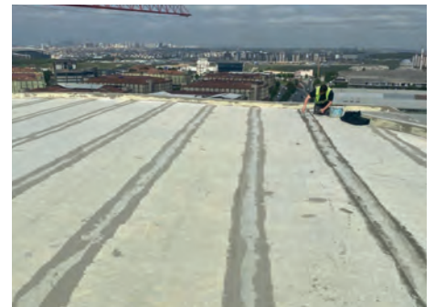
Waterproofing of 35.000 m 2 of DRY120 in all its outdoor walkable terraces. PENINSULA SHOPPING CENTRE. Tijuana. Mexico.
