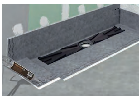
14. Apply a strip of REVESTTECHFLEX adhesive before overlapping the membrane of the rest of the shower.
