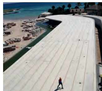
Waterproofing of 8.000 m 2 of flat wakable roofs with DRY80 . Hotel SAINT REGIS Punta Cana. Dominican Republic.
