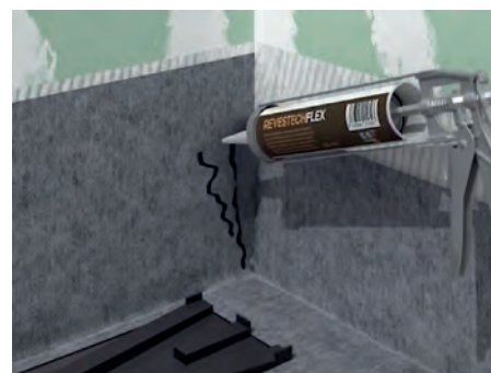
13. Form the corners by folding the membrane. Apply REVESTTECHFLEX to adhere the fold.
