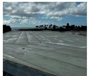
Waterproofing of 8.000 m 2 of flat wakable roofs with DRY80 . Hotel SAINT REGIS Punta Cana. Dominican Republic.
