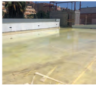
Waterproofing of terraces with DRY80 . SHOPPING CENTRE EL SALADAR_ Fuerteventura (Las Palmas).
