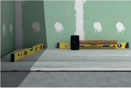
INSTALLATION OF THE SHOWER TRAY
