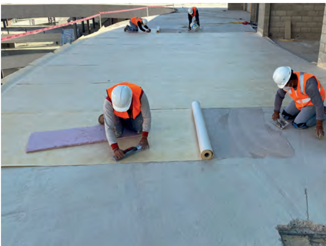
Waterproofing of 35.000 m 2 of DRY120 in all its outdoor walkable terraces. PENINSULA SHOPPING CENTRE. Tijuana. Mexico.
