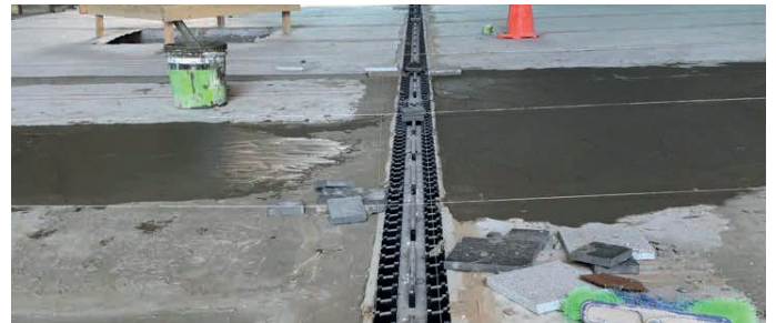
Waterproofing of 18.000 m 2 with DRY120 and drainage with WALK LEVEL . RESIDENTIAL AND COMMERCIAL PROJECT URBANA APOQUINDO. Santiago de Chile.
