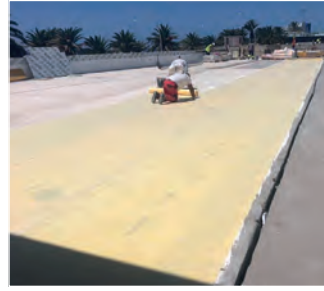
Waterproofing of terraces with DRY80 . SHOPPING CENTRE EL SALADAR_ Fuerteventura (Las Palmas).
