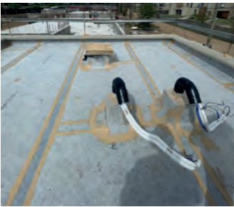
Waterproofing of walkable flat roofs with ECODRY120 . RESIDENTIAL SINGLE-FAMILY HOMES. Montevideo. Uruguay.
