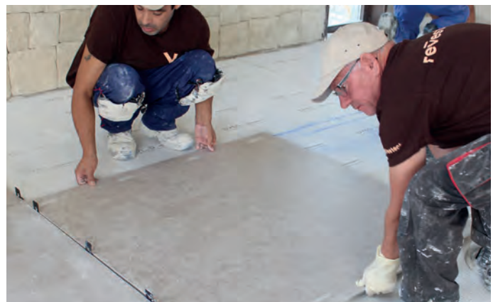
6. Before installing the tiles, wait at least 24 h. for the adhesive on the membrane to dry. Use the adhesive recommended by the manufacturer of the tiles to adhere them to the membrane.
