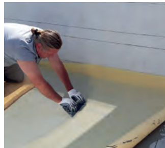
Waterproofing of terraces with DRY80 . SHOPPING CENTRE EL SALADAR_ Fuerteventura (Las Palmas).
