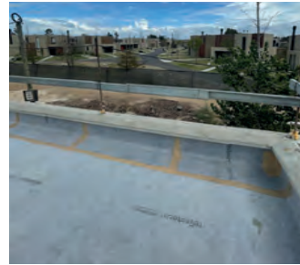
Waterproofing of walkable flat roofs with ECODRY120 . RESIDENTIAL SINGLE-FAMILY HOMES. Montevideo. Uruguay.
