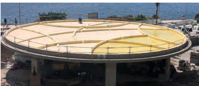
Waterproofing with DRY80 of the pool bar roof of the 5-star resort CHAIN H10_Costa Adeje (Tenerife).
