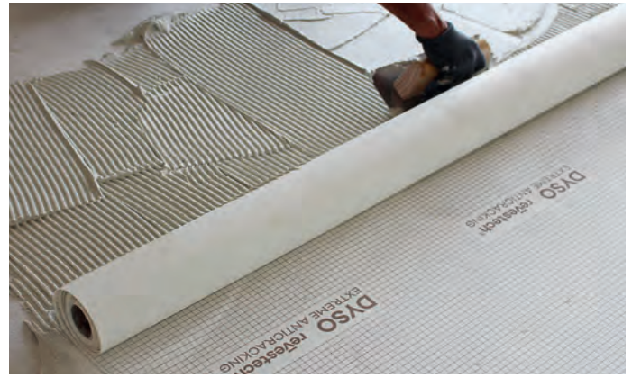
2. Apply C2 S1/S2 tile adhesive with a 4/6 mm notched trowel. Apply the adhesive on small patches to prevent drying and always in the same direction. Do not install the DYSO membrane on semi-set adhesive.
